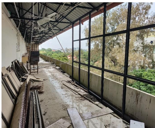
Picture 4.1: Sidewalls blown away and glass panels broken to pieces at Pareeksha Bhavan, 16 October 2018
