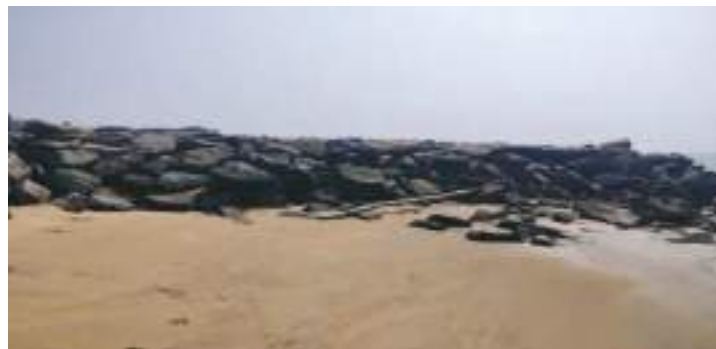
Fig.16 A view of the damaged groyne Aniyal beach Edavanakkad Grama Panchayat (South)
