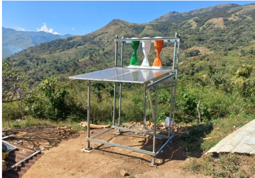
A Typical 1.5 kW Solar Wind Hybrid System installed in Melethudukki
