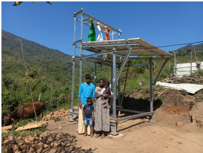
A Typical 1.5 kW Solar Wind Hybrid System installed in Melethudukki
