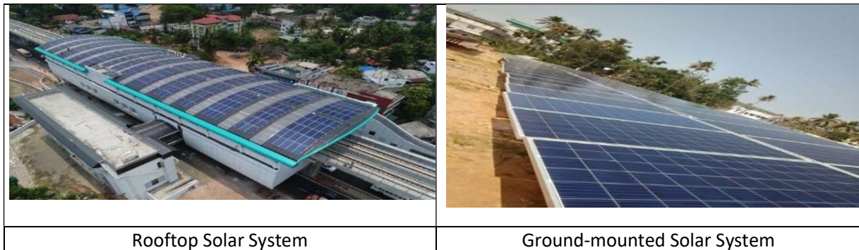
Mounting arrangements of solar panels in roof top and Ground
