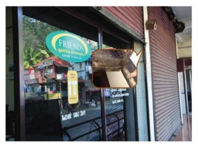
Picture depicts view of Idukki Centre, where the steel shutter cannot be closed. The shutter channel is blocked with wooden logs to prevent collapsing of the damaged steel shutter. Inset picture displays a wooden log used as blockade.
