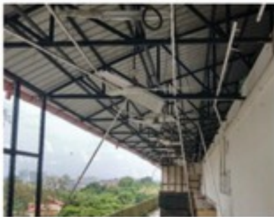
Picture 4.2: Remnants of false ceiling hanging from the roof at Pareeksha Bhavan, 16 October 2018
