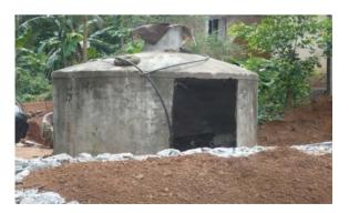
the well constructed by the GP or from nearby streams. The beneficiary HHs stated that the RWHS were not used for collecting since water inception, due to leakages in tank. The installation of RWHS in areas where conventional WSS were feasible and defective construction including non-installation of filter units led to failure of scheme. Government stated in the Exit Conference that the issue will be examined.
