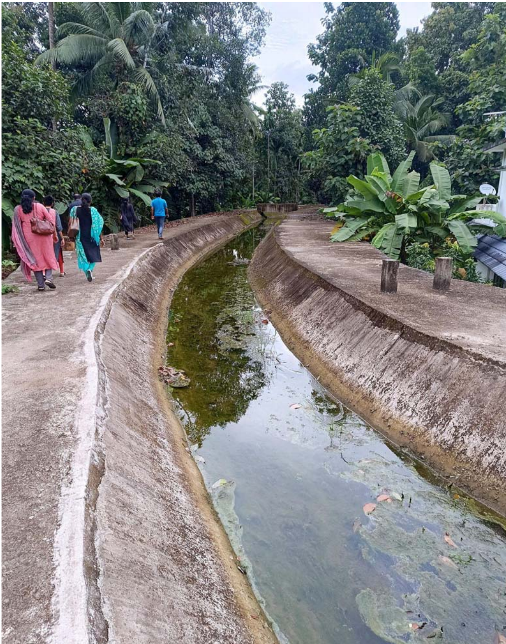
Photo 2.1 : Urgent rectification works at the breached portion of Kadappoor distributary from ch 1410m to 1505m
