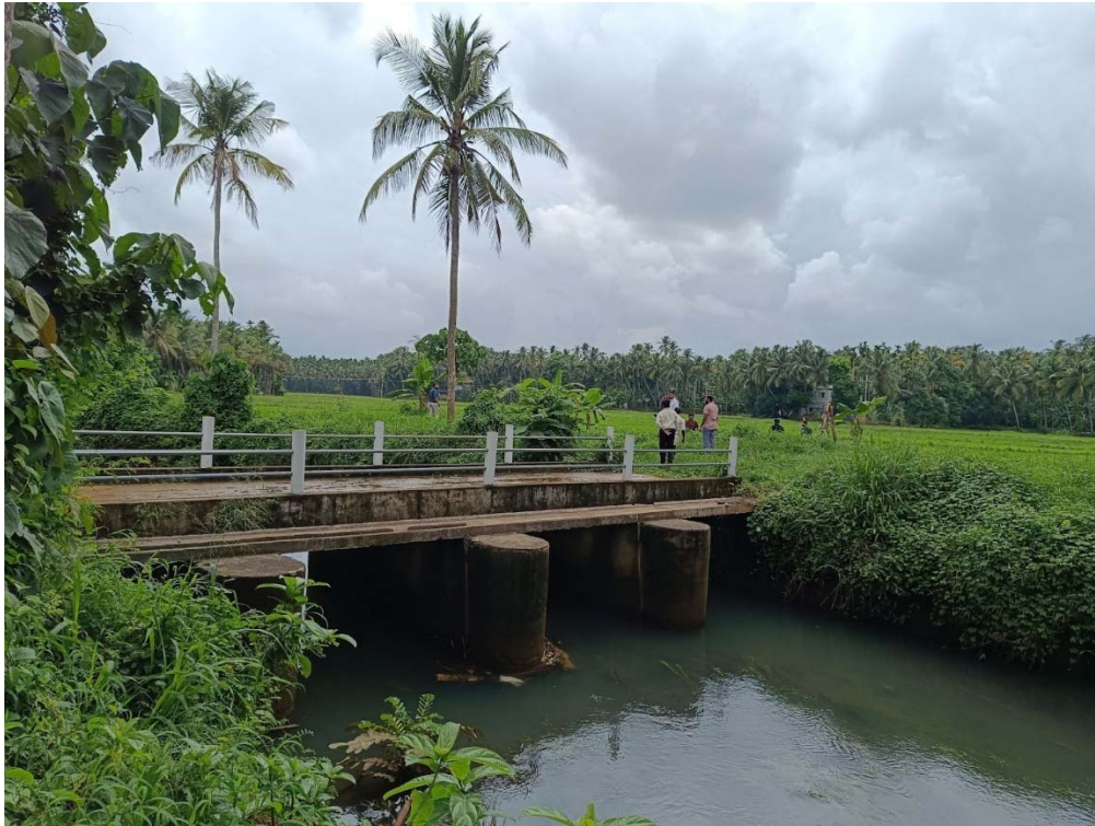
Photo 2.5: Construction of VCB with tractor slab across Kooriyad thodu at Ayyankolypadam in Kottakkal Municipality in Malappuram District
