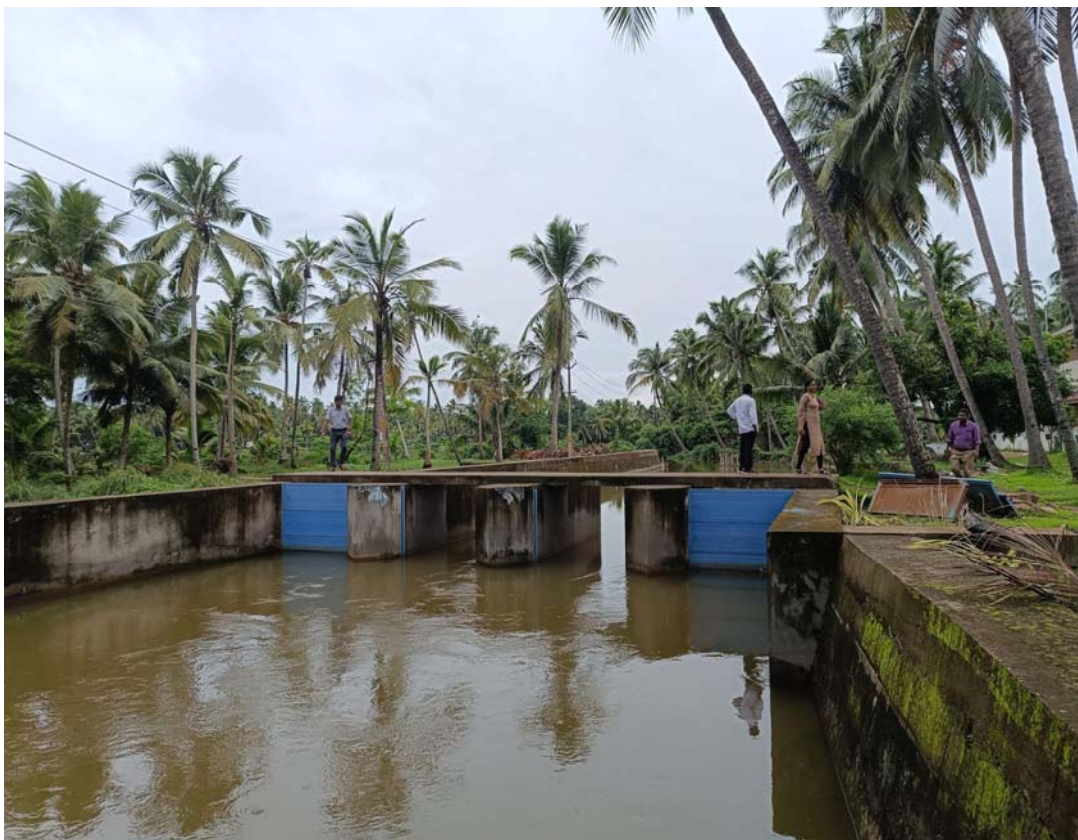
Photo 2.4 : Construction of SWE VCB across Madathil thodu at Kanchiramukku in Maranchery Grama Panchayat in Malappuram.
