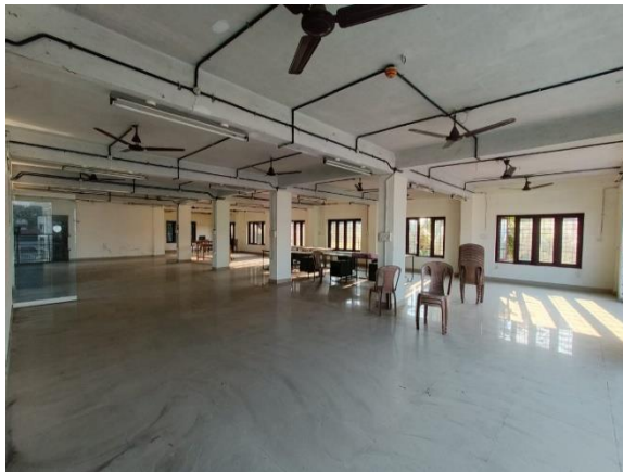
Figure 5.1: Floor 2 of BOCWWB Ernakulam District Office building, Edappally not rented out and lying vacant. Photo taken by Audit Party on 11 October 2023
