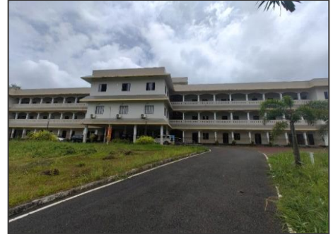
Figure 5.5: Unauthorised construction at SN College of Advanced Studies in Varkala Municipality
