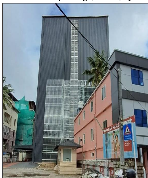
Figure 5.8: Multi-level mechanised car parking in Kalyan Silks at Kochi Corporation
