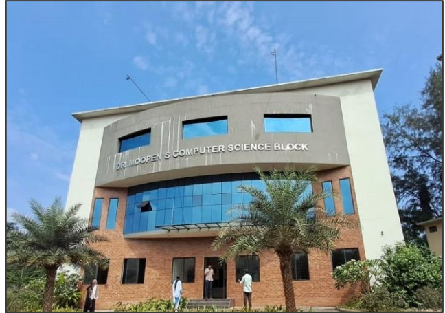
Figure 5.7: Unauthorised construction at Farook College in Ramanattukara Municipality
