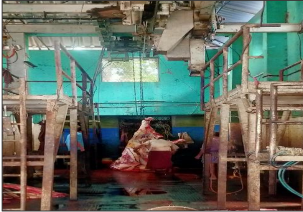
Figure 7.1: Corroded machinery, cutting of meat from Carcass partially touching the floor
