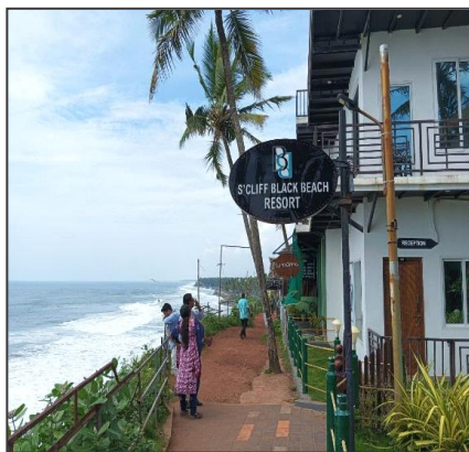
Figure 5.3: Black beach resort constructed in CRZ area within 10 meters from cliff in Varkala Municipality
